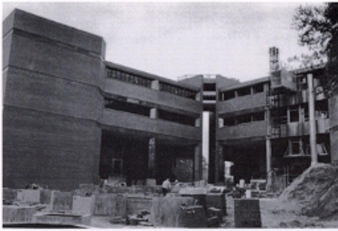
The CSE building, under construction in the mid-80s.
